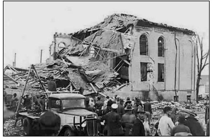
New London School Building After Gas Leak Explosion
